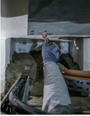
NuPLUG 1120 is a mortar used as a radiation and fire barrier in the sealing of penetrations, mainly in nuclear power plants or other nuclear sites.
