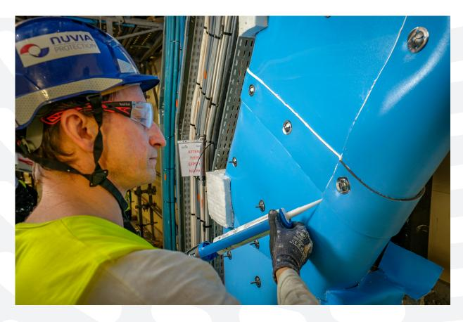
NuFLS 5810 is a product that provides the heat load subtraction function from the heat load of cables from certain fire initiations, acting as a fire initiator creating a thermal barrier effect. This product is to be used when the cables are outside the fire plume of the fire initiator
