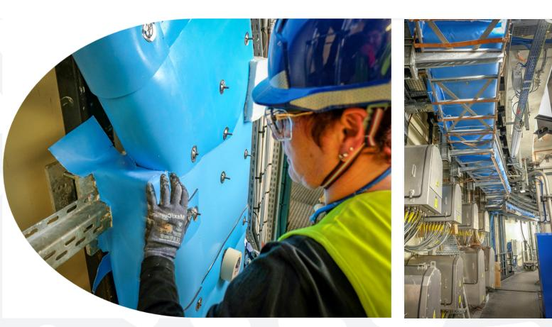
NuFLS 5100 is a flexible protection, which aims to reduce the heat load of a fire volume. This protection allows the heat load of a set of cables to be subtracted and avoid the aggravation in the event of a fire, thus safeguarding the surrounding technical equipment
