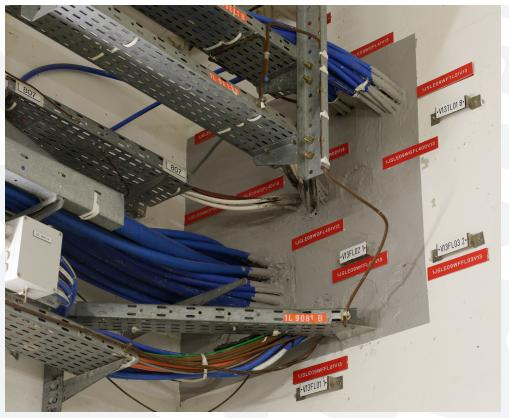
NuCOAT 3110 is a silicone elastomer used as a surface coating to protect or repair surfaces with high sealing requirements (water, air) or specific requirements (decontaminability, resistance to aggressive liquids, etc.)
