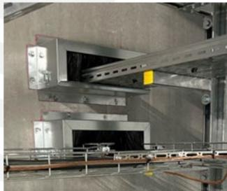
The NuPLUG\_I04 a fire-resistant cable box for the caulking of electrical cables.
