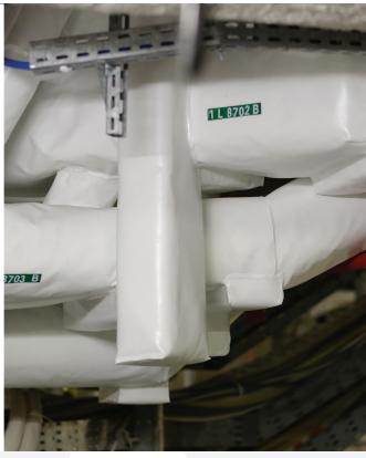
NUVIATech Protection, brand of NUVIA Group, offers various protection products for electrical systems. Products intended for the fire zoning through antipropagation systems such as flame screens or mats for cable trays or cable shafts. Products for maintaining the functionality of electrical systems through rigid enclosures or flexible wrapping around cable trays.
