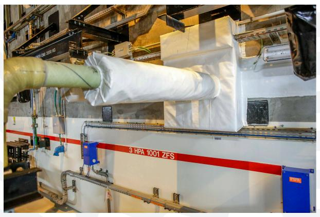
PlugPART 5110 is a multicomponent fire barrier complex, used for sealing of electrical, mechanical crossings, blank and mixed on walls or slabs
