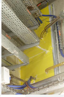
NuPLUG 3110 is a silicone elastomer used as a waterproof fire barrier in the sealing of penetrations, mainly in nuclear power plants or other nuclear sites.
