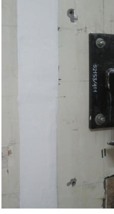
NuJOINT 3120 is a complex of mineral wool, refactory adhesive and silicone elastomer used as a fire and waterproof barrier in the sealing of interbuilding joints, mainly in nuclear plants or other nuclear sites, or any other industrial site.
