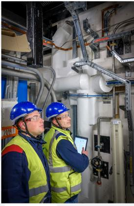
NuFCT 5110 is a flexible protection, ensuring functionality of the protected cable tray for up to 2 hours under ISO. It is adaptable to the environment. This protection is composed of mineral wool, refactory adhesive and a protective fabric. This complex has a thickness of 80mm.
