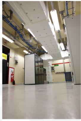
NuDUCT 5190 is a flexible protection, providing up to 3 hours of protection depending on the configuration. It is adaptable to the environment. This protection consists of mineral wool, refractory adhesive and a protective fabric. This complex is 80 mm thick.
