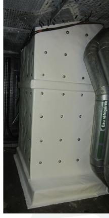
NuDUCT 5111 is a flexible protection, providing protection for up to 3 hours depending on the configuration. It is adaptable to the environment. This protection is composed of mineral wool, refactory glue and a protective fabric. This complex has a thickness of 80 mm.
