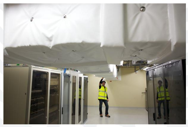
NuDUCT 5110 is a flexible protection, ensuring protection up to 2 hours, depending on the configuration; It is adaptable to the environment; This protection is composed of mineral wool, glue refactory and a protection fabric; This complex has a thickness of 80 mm.
